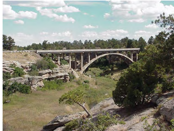
Cherry Creek Bridge, Douglas County, Rehab
