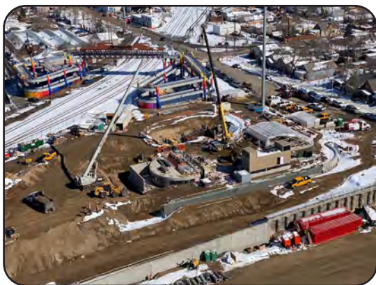
Image 16. Aerial of Pump Station near York Street
