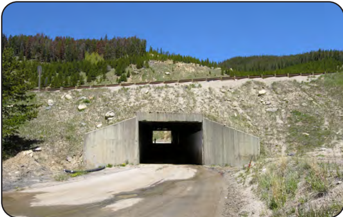
Image 7. I-70 over Forest Service Rd (F-13-S_Minor)
