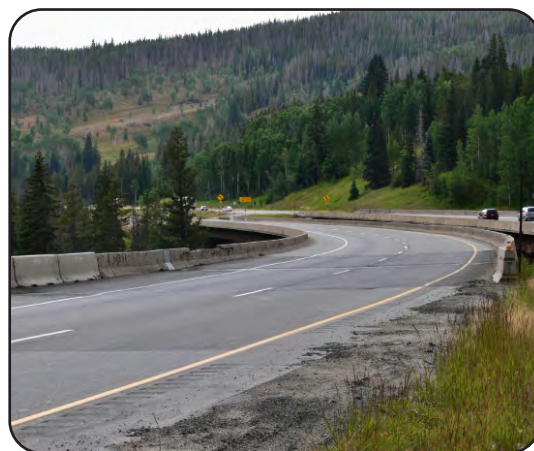
Image 21. I-70 over Polk Creek in Eagle County (F-12-AS)
