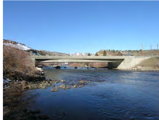
Structure F-10-AH, (Wolcott)
