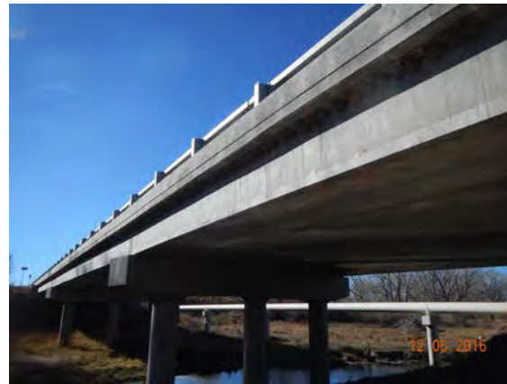
O-19-R (Purgatoire River Bridge)
