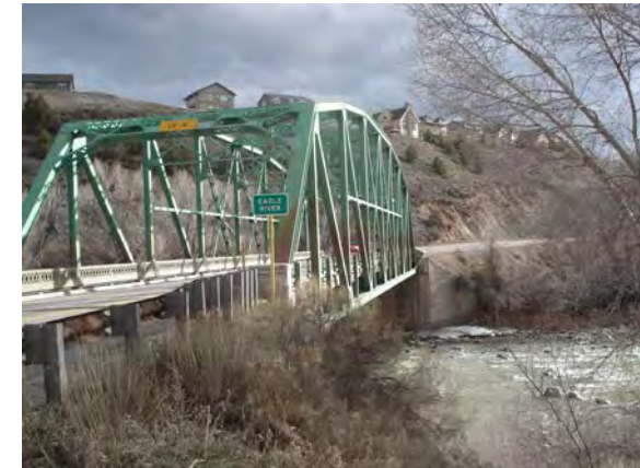
Eagle River Bridge, Eagle County, 2012
