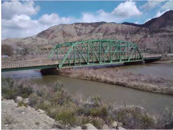
Dotsero Bridge, Eagle County, 2013
