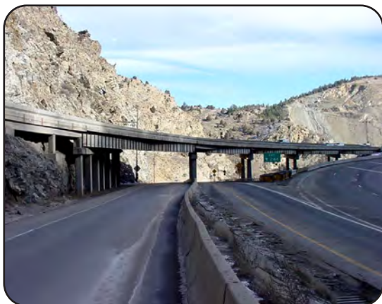
Image 20. I-70 over US6 and Clear Creek in Clear Creek County (F-15-BL)
